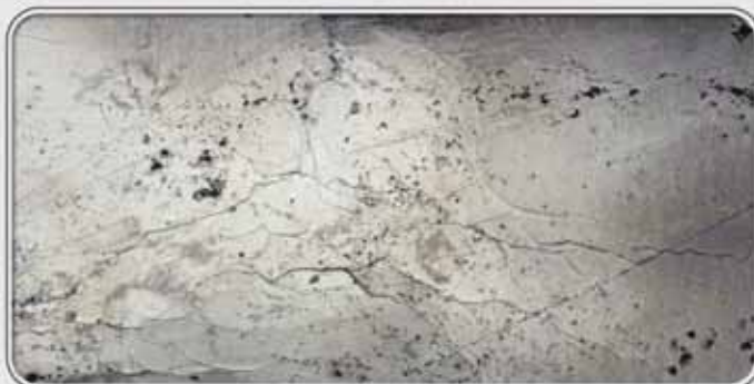
Picture of 304 stainless from actual outdoor wood furnace
