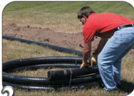
3 Place ThermoPEX into trench.
